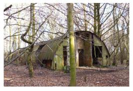
The Nissen Hut could be packed in a standard army truck and erected by six men in four hours. The world record for constructing one is 1 hour 27 minutes.
